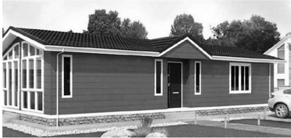
*Park Homes are of light construction, typically transported on two trailers and then assembled.*
