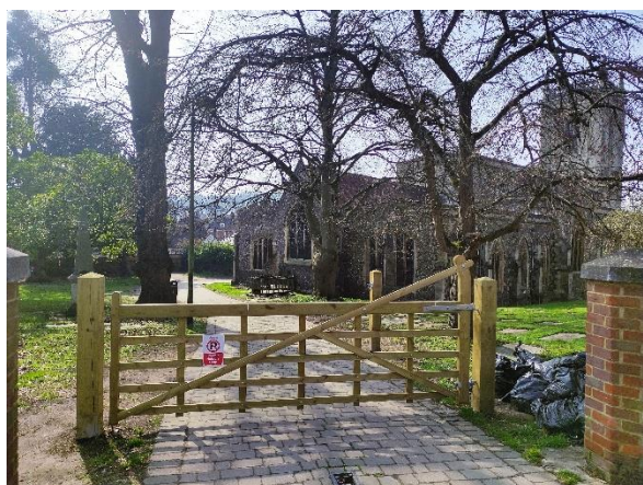
The Good: a sturdy gate to deter unauthorised access.
