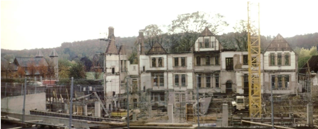
In 1990 the original former Tech's school buildings were demolished, keeping only the Vernon façade. This scene of work in progress was captured in a documentary called "Wycombe World 1990" by John Smithson of the High Wycombe Film Society. The film can be viewed on YouTube (see p14).
