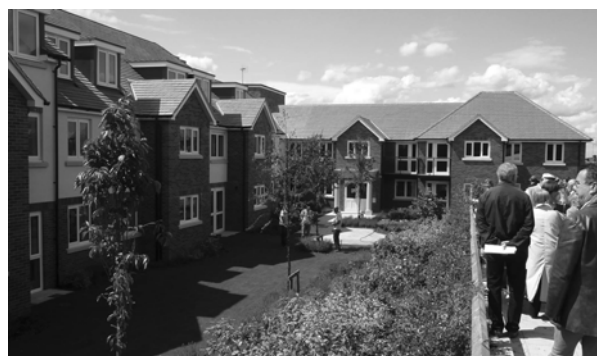
Windsor Lodge, Princes Risborough. Car-owning discouraged.
