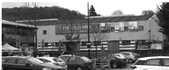
Site of the proposed Aldi Store in Tannery Road viewed from across the Halfords car park
