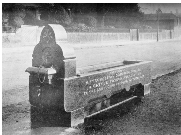
The Trough opposite Park House on the London Road Photo courtesy London Metropolitan Archives
