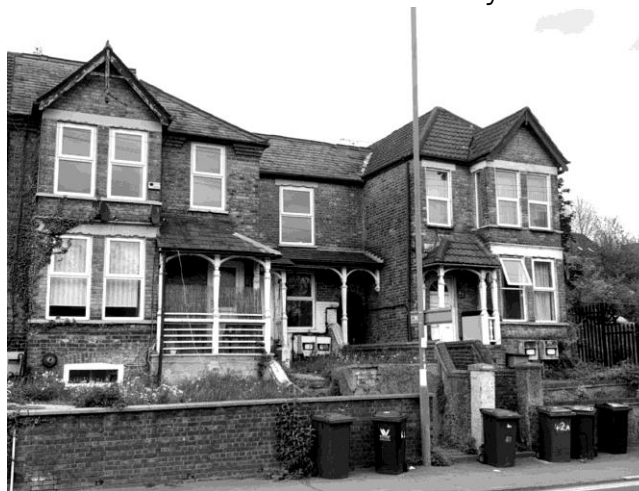
Houses on West Wycombe Road before demolition
