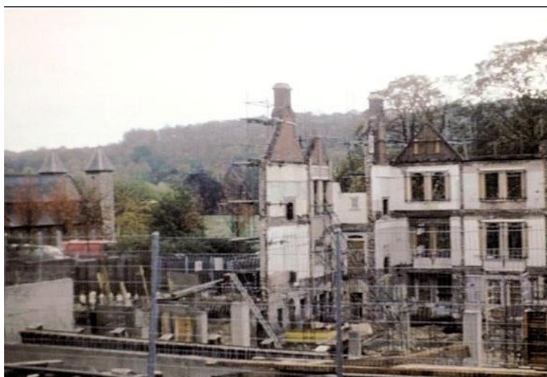
A 1990 documentary in the SOFA collection captured the scene from Railway Place when only the façade of the old Grammar School buildings remained held in place by scaffolding.
