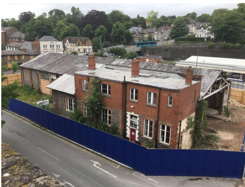
Refurbishment in progress at the Brunel Shed viewed from a vantage point in the multi-storey carpark – Photo Chris Woodman
