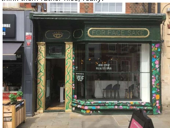
12 High Street was once part of the Antelope Inn and still retains some eighteenth-century architectural features. Should a shopfront policy encourage or restrain such cheerful embellishments? Photo: Chris Woodman
