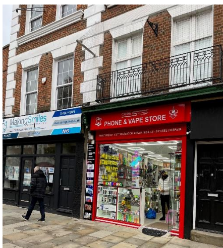
The red colour at No.8 High Street does not fit in with the colours of the Conservation Area, while next-door, the "Making Smiles" fascia nameboard does not fit with the traditional timber front.
