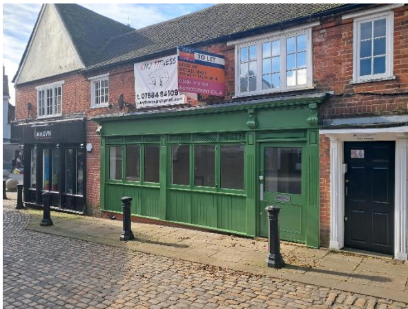
A sympathetic restoration with a shopfront that Planning Group support
